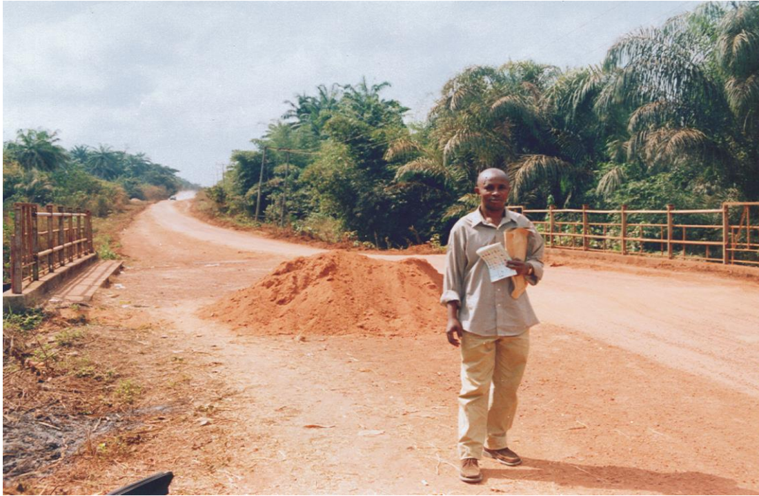
One of the researchers on top the Eze Bridge at Amaneze; the bridge links Ugwuoke to Alayi, Isiukwuato, Ohafia, etc., built by the indefatigable Ugwuoke women.
